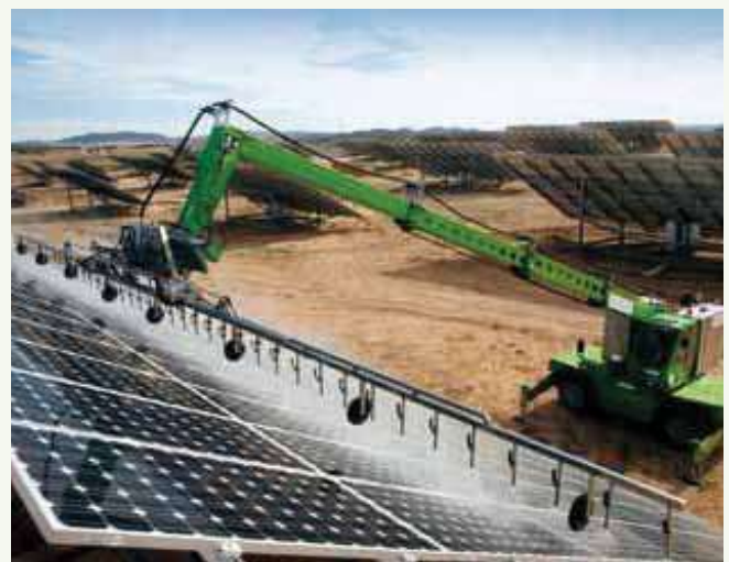
Figure 24: Module Cleaning Using Crane
