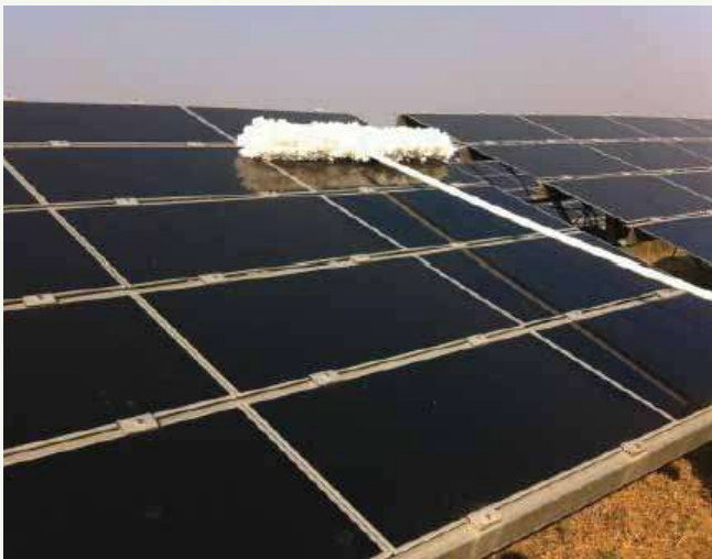
Figure 26 : Module Cleaning Using Dust Broom
