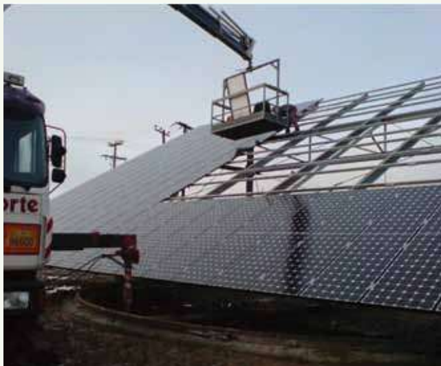
Figure 23: Module Installation on a Large Tracking System
