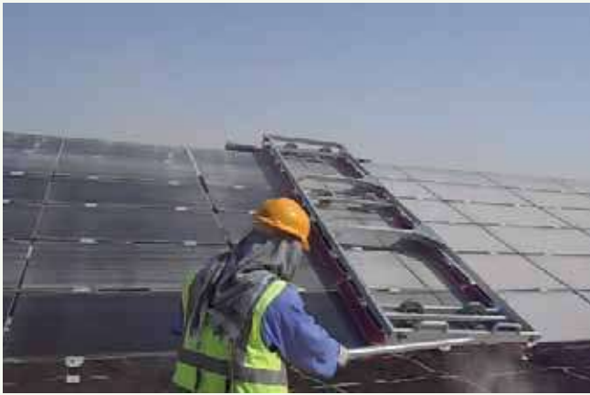
Figure 25: Module Cleaning Using Brush Trolley
